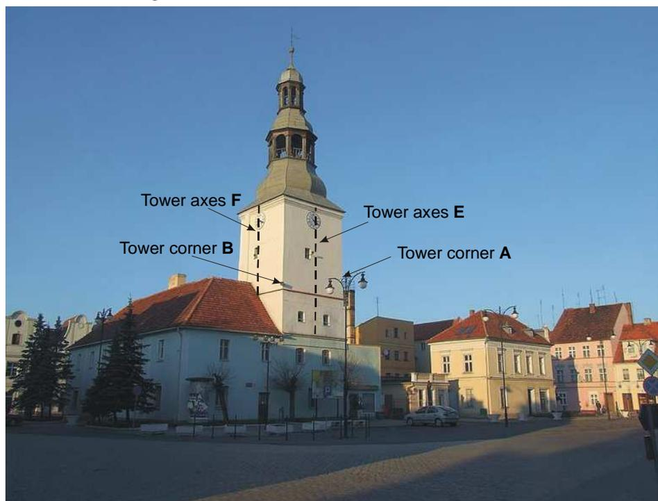
Fig. 1. Tower corners and axes subjected to measurements
