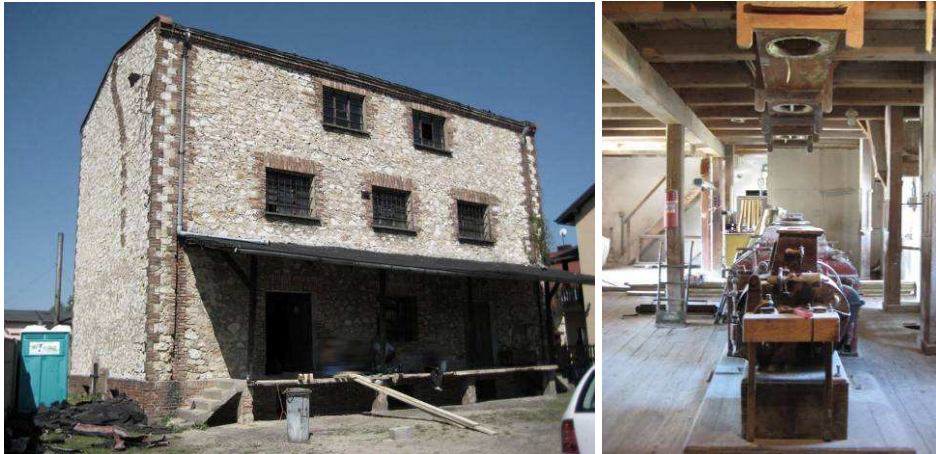
Photographs 1, 2. Młyn Zygmunt (Zygmunt Mill) Restaurant building prior to renovation, (photograph by A. Grzonka, 2011)
