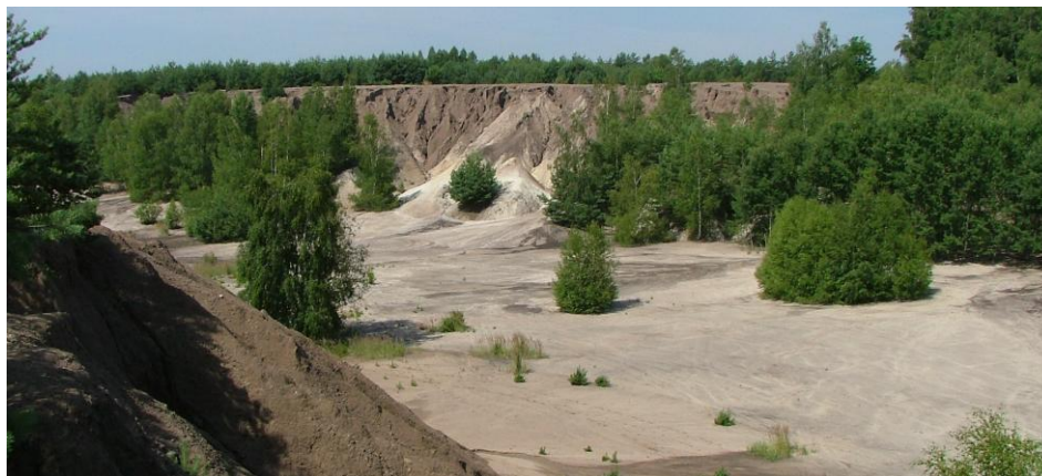
Fig. 2. A view on reclaimed area 20 years after leveling and slopes forming. The strong erosion processes (ravine erosion) are observed
