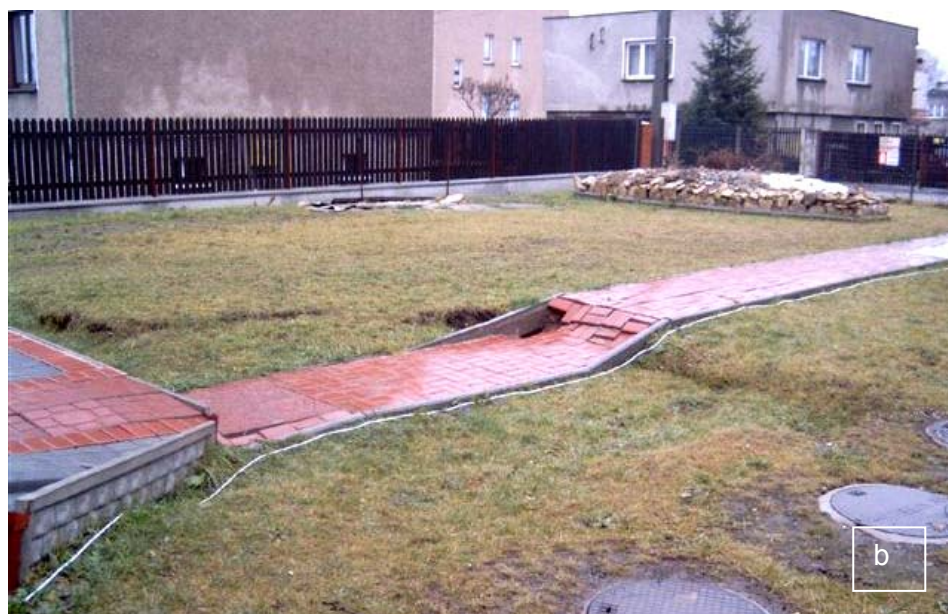
Fig. 2. Vertical fissure (a), and a surficial scarp in an urban area (fot. K. Szafulera)
