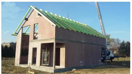
Fig. 6. Two-storey house in Wyry - installation of the roof; authors' own photographs
