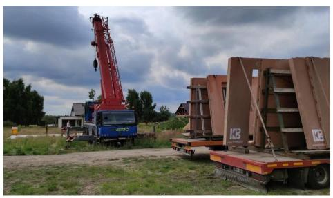
Fig. 2. Expanded clay concrete panels, authors' own photographs
