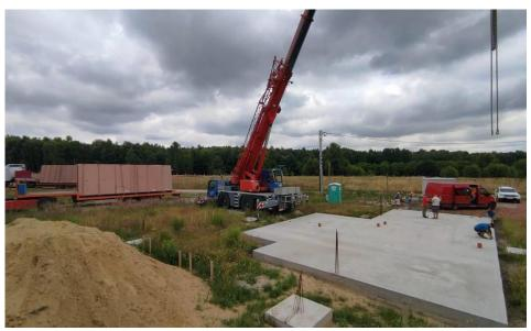
Fig. 4. Two-storey house in Pilchowice, concrete foundation slab and installation of prefabricated walls is started, authors' own photographs
