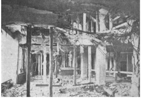
Fig. 4. Damage caused by the German bombing in September 1939. An entire span and part of the floor is missing [4]
