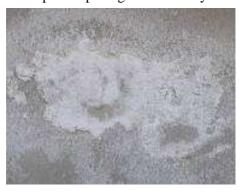
Fig. 1. Surface crystallization-wall and plaster remain overdamped
