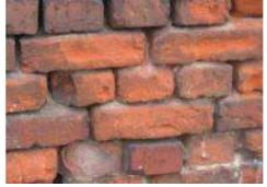
Fig. 3. Effects of corrosion with cement mortar stronger than ceramic material
