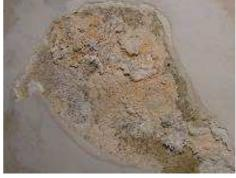
Fig. 2. Crystallization of the salt within the plaster
