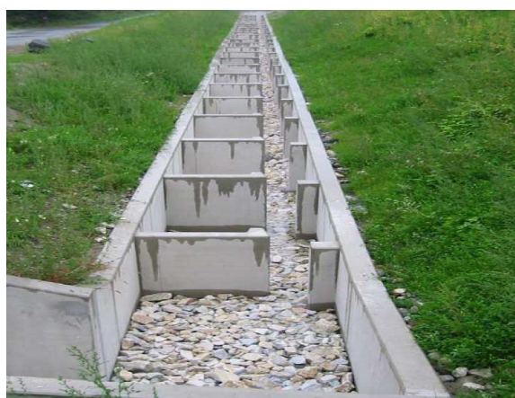
Fig. 2. Vertical slot fish pass by Villach/Austria [9]
