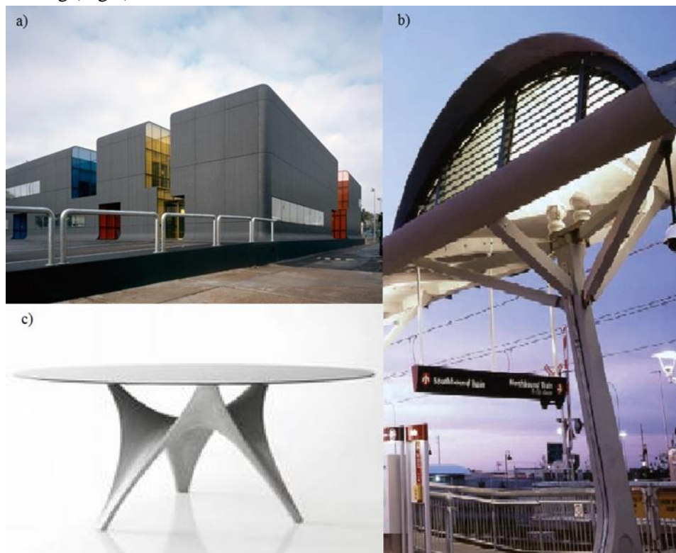
Fig. 1. Examples of applications of reactive powder concrete [9]: a) elevation of the Bus Centre in Thiais France, b) roofing at the railway station in Calgary, c) a table
