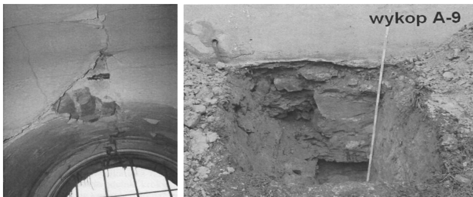
Fig. 3. Lintel with a visible crack exposing the reinforcing steel, 5 th floor (tower) [4].
