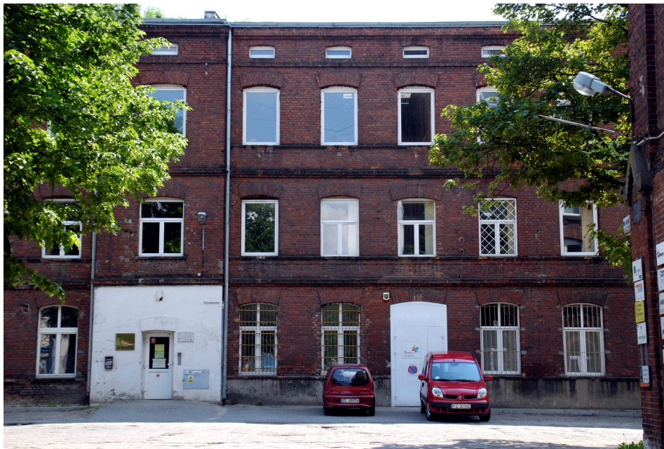
Fig. 4. An example of a building where an uncontrolled replacement of window frames led to the complete loss of the original aesthetics. Photo A. Kurzac
