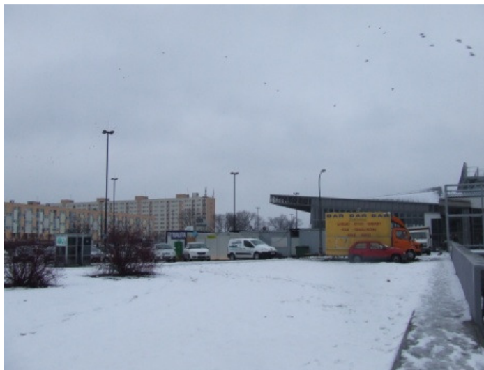
Fot. 1. Teren zielenca tranzytowego przy Dworcu Wschodnim; widok na budynek dworca [Domanowska 2012] Phot. 1. Transit area covered with lawn at the East Railway Station; view on the building of station [Domanowska 2012]
